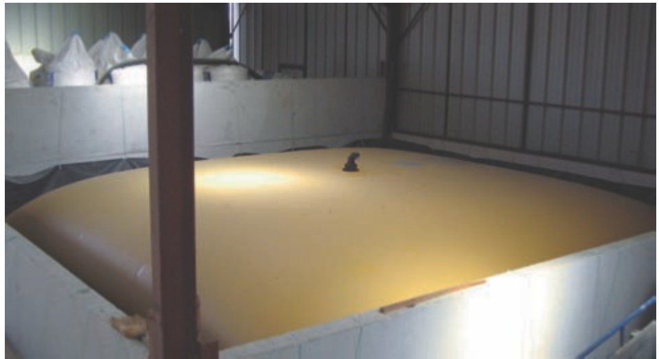
50m 3 nitrogenous solution with internal retention basin
