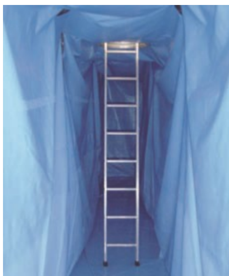
Ship slipway leakproofing
