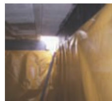
Old tank leakproofing
