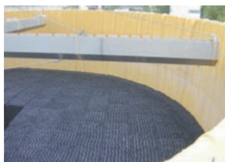
Concrete tank leakproofing
