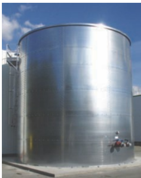
Bolted tank with PVC liner
