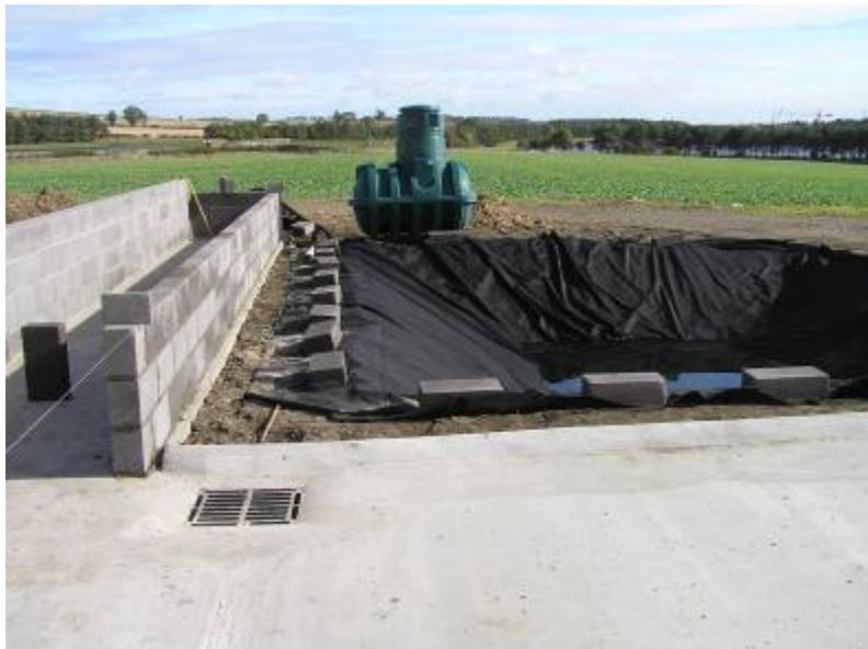
**Indirect biobed system under construction.** Bunded handling area in foreground, with a boom wash out section all draining to single collector. Background - hole waiting to be filled with biomix and secure intercept tank awaiting installation.
