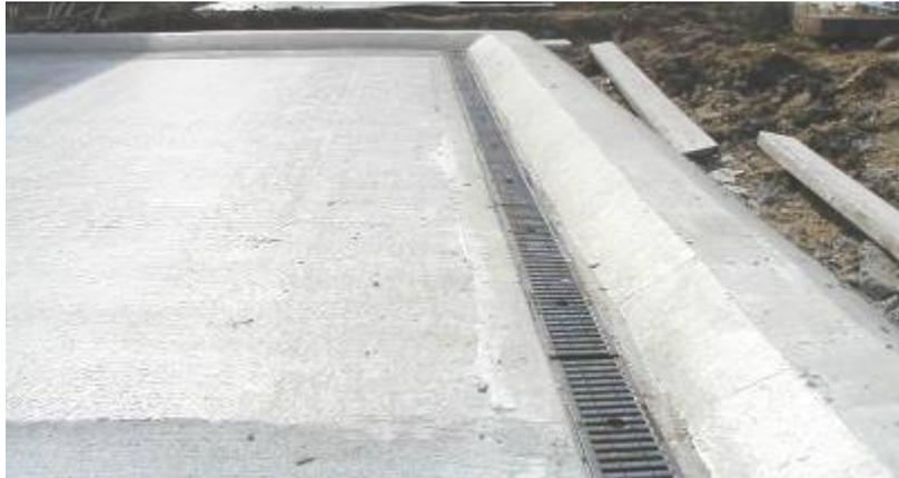
**Concrete pesticide handling area with bund and ACO type drainage system**
