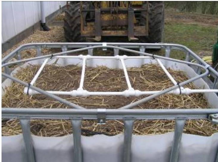
Plate..... Distribution pipe work above each IBC
